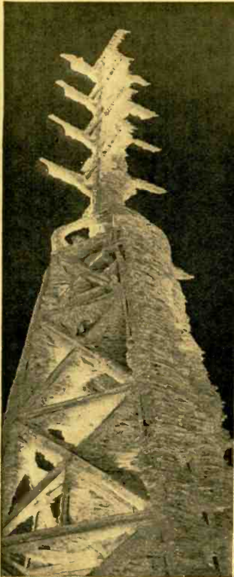
Left: Ice-covered mast of the Yankee Network's FM Station W39B, Mt. Washington. Tons of these ice feathers are continually forming on all exposed surfaces. Right: Another view of the antenna of W39B, Mt. Washington, showing peculiar auto-spring construction of antenna arms. They are constructed to stand the weights of tons of ice.
