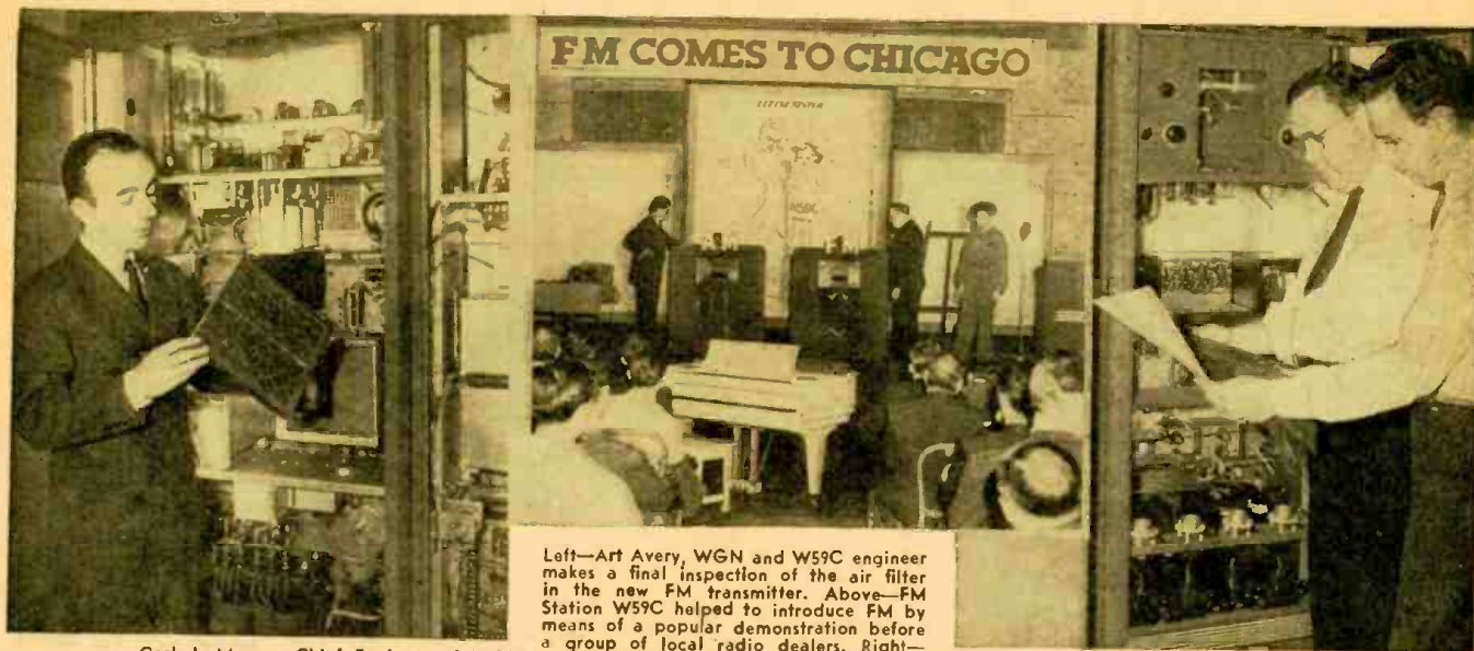
Left—Art Avery, WGN and W59C engineer makes a final inspection of the air filter in the new FM transmitter. Above—FM Station W59C helped to introduce FM by means of a popular demonstration before a group of local radio dealers. Right—Carl J. Meyers, Chief Engineer of WGN and W59C (left) and his Assistant, Clyde White, during installation of FM transmitter.
